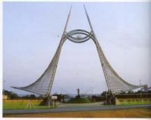
Designed by Delhi-based Kamath Design Studio, the gateway is 33m high, weighing approximately 20 tonnes. It is the tallest Stainless Steel (SS) structure in South Asia, erected of straight SS pipes, and forms the entrance to Jindal Steel and Power Limited at Raigarh in Chhattisgarh.
