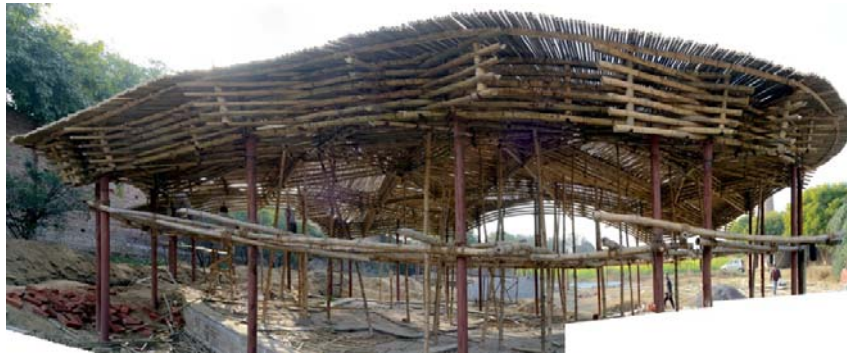
Figure 6. The woven bamboo permanent formwork ready to receive the bamboo-crete.
