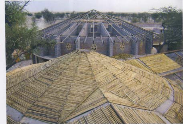
The 'neo-jhumpas' boast of an articulated triangulated steel frame that holds up a bamboo roof finally decked out in concrete. Above: A layer of soil and grass imparts thermal mass to the roof, thus lowering indoor temperatures
