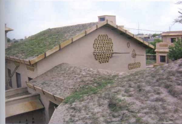
The buildings sport a graft of stonework that has added a layer of 'localisation' as well as functioning as 'vents' to ensure pressure equalisation during frequent dust storms
