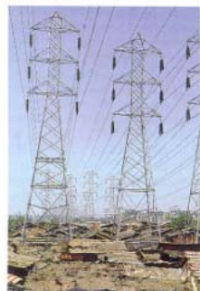
A contradictory perception of security. Miles of hutment under high tension wires represents a highly dangerous housing location as perceived by the planners, city fathers and the casual observer. But, for those who have chosen to live here, this constitutes the most secure location — perhaps the last one to face a demolition threat as it has no real estate value.
